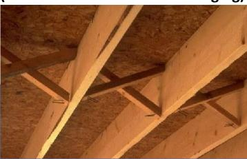
Transfers the floor loads to adjacent joists
